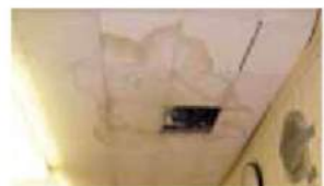
Result w/ Fibrous: Mold growth on ceiling from water drip (corrosion on duct also possible)
