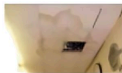
Result w/ Fibrous: Mold growth on ceiling from water drip (corrosion on duct also possible)
