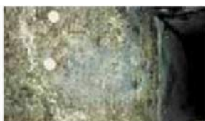
Result w/ Fibrous: Mold growth on insulation
